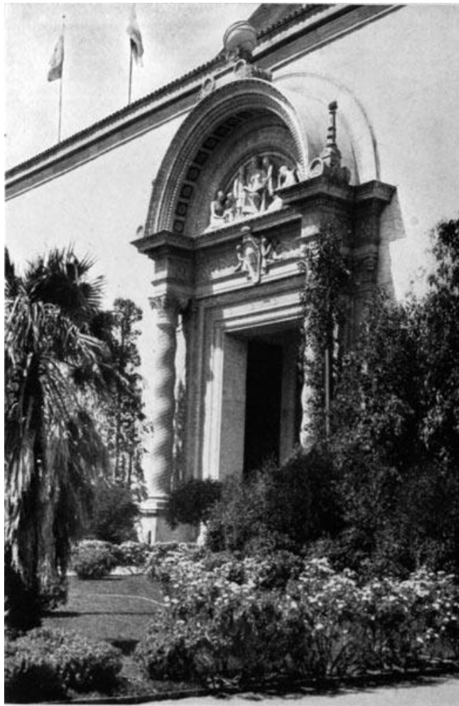
Palace of Education Main South Portal
